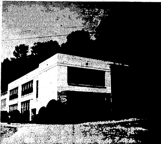
Grade School Being Repainted
