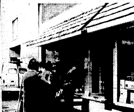
The old Stadman building, now owned by Mike Walston, was given the first part of a remodeling job to match it up with the adjoining buildings on the sunny side of the street. Tim Roetman and crew did the carpentry.
