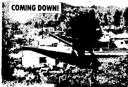
Old Prater home in Mill Addition being removed as part of local Clean-Up drive. Other vacant houses slated for similar treatment to rid town of eyesore of abandoned homes.
