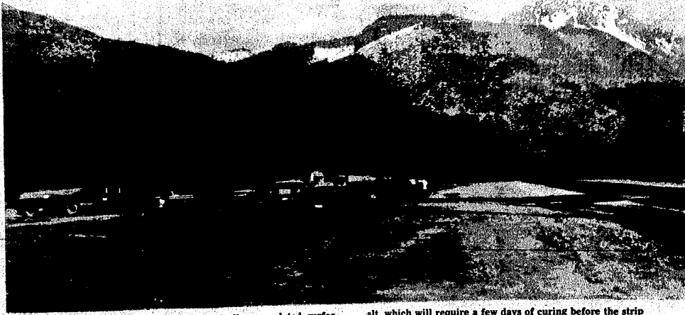
Snelson Company of Sedro-Woolley completed surfacing of the Concrete Airport on Monday of this week. The soil-cement paving was topped off with a seal coat of asphalt, which will require a few days of curing before the strip can be used. The runway has been lengthened and a taxi strip and parking area given a hard surface treatment.
