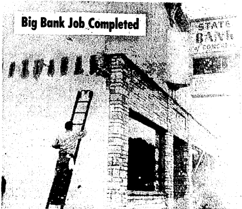
Roy Pyatte, working with contractor Andy Thompson, puts the finishing touch on the big job of repainting the bank building. It is now a pleasant gray—top to bottom, back and sides.
