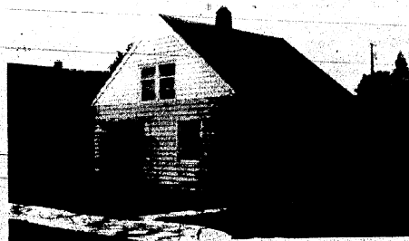
In Mill Addition the C. S. Phillips rentals are being given a new touch of color. This home is occupied by Peggy Landsaw and is now a neat turquoise and white.
