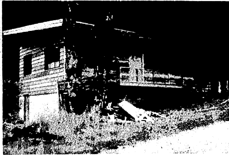
A building on Seidel St., started many years ago and never completed, is now shaping into a fine modern addition to Concrete's residential inventory. The new home belongs to Mr. and Mrs. Bob Reidy of Oak Harbor, who plan to make their home here soon.
