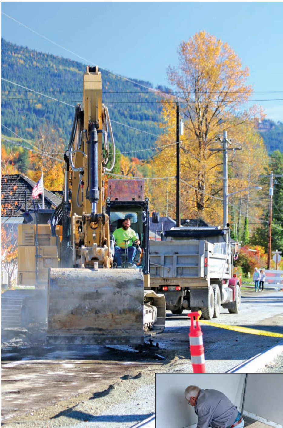
Above: A Trimaxx Construction worker uses a CAT 335 to scrape away the failed top layer of asphalt on W. Main St. in Concrete, in preparation for repaving the roadway in late October and early November. The street restoration project stretches from Superior Ave. N. to Grasmere Rd., and also reclaims the original neighborhood fabric, complete with safer, walkable sidewalks and alley access for some residents. Trimaxx is picking up its pace to complete key weather-reliant components of the project—including asphalt-laying—before winter rains begin in earnest.
