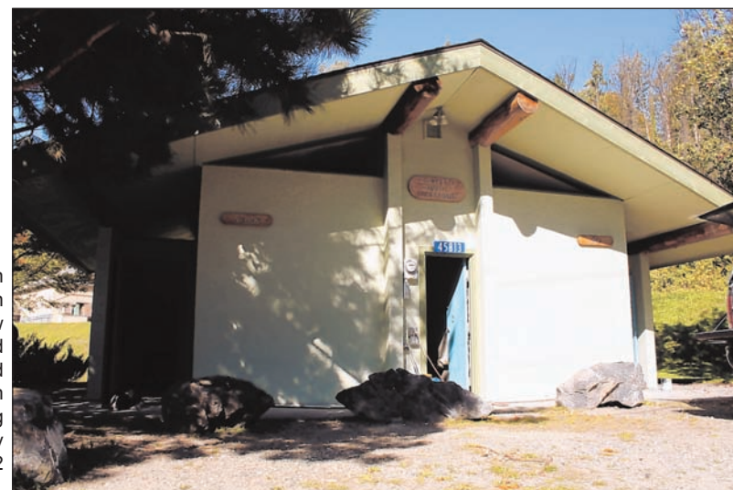
Right: The public restrooms on Main Street in Concrete got a thorough renovation. Upgrades included a new roof and skylights; painting inside and out; new sheetrock, insulation, and Plexiglas windows; and teak oil on the exposed logs. "I'm glad to hang my hat on this project. It looks really good," said Jack McCormick, M2 Construction owner/operator.
